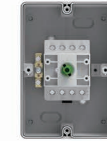
防水盒安装 Waterproof box installation
